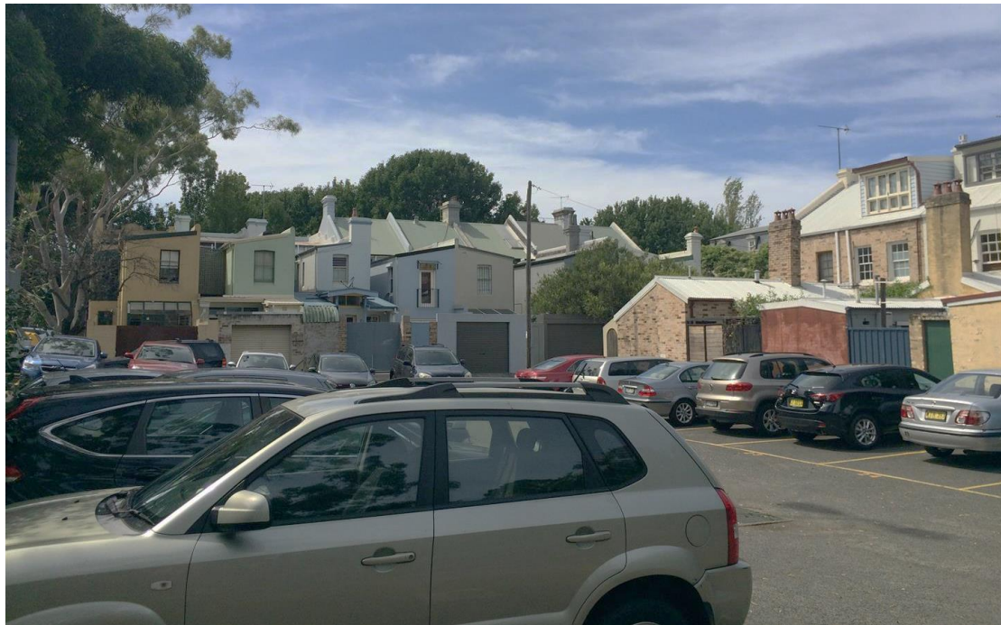
Figure 14: View looking south-east across the car park to existing two-storey terraces fronting Baptist and Boronia Streets
